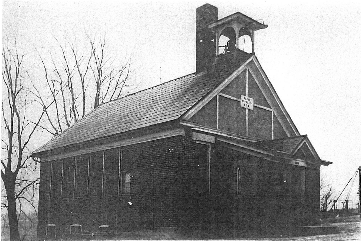
Photo No. 7 - High Street School - 1952
