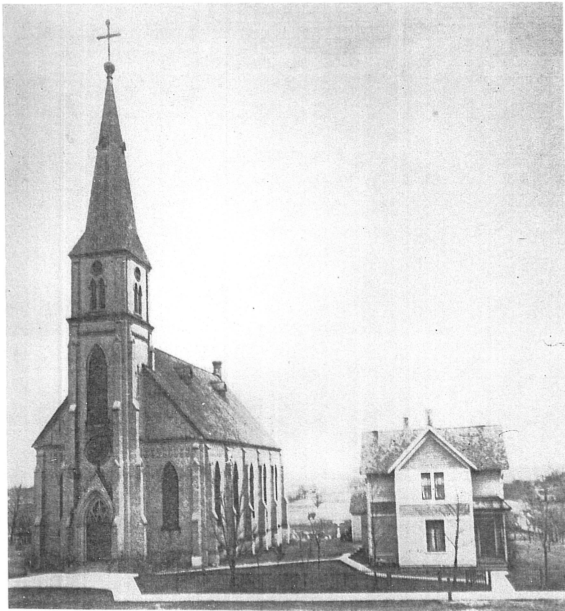
Photo No. 27 - Second St. Alphonsus Church and Parsonage Burned 1906
