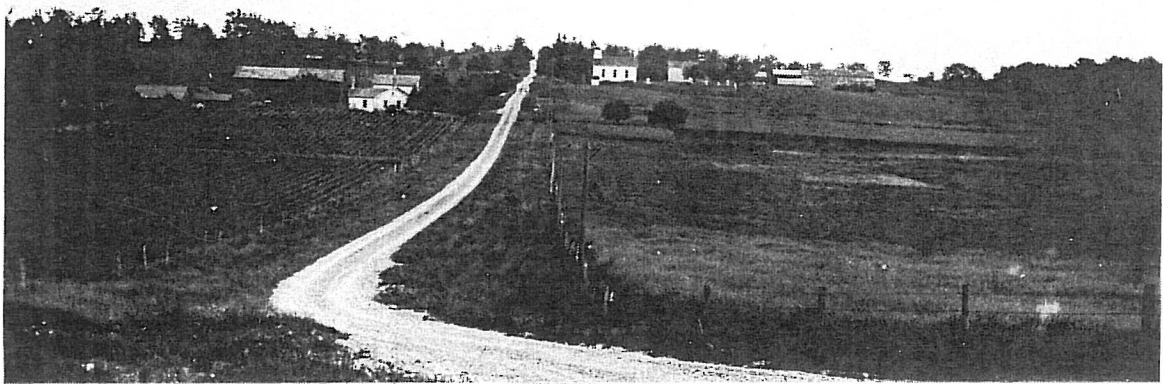
Photo No. 15 - High Street Road - About 1913
