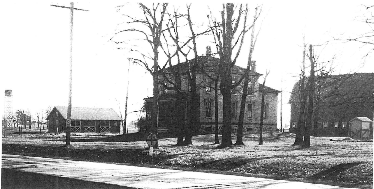
Photo No. 10 - Oakwood Shores Prior To Railroad Overhead
